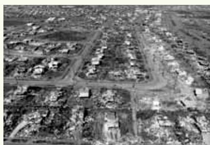
Above: The aftermath of Cyclone Tracy, 1974.
