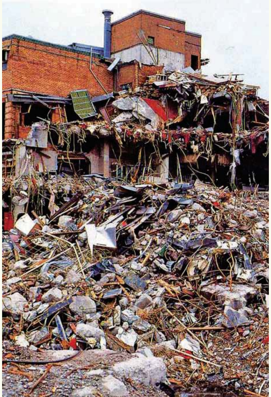
Above: The Newcastle Workers Club after the earthquake.
